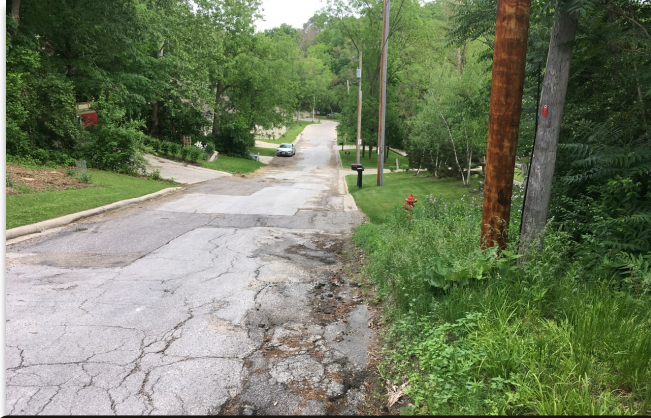
Undergrounding Existing Aerial Utilities
