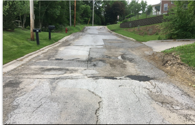
Repave North Gilbert Street
