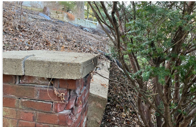
Addressing Retaining Walls
