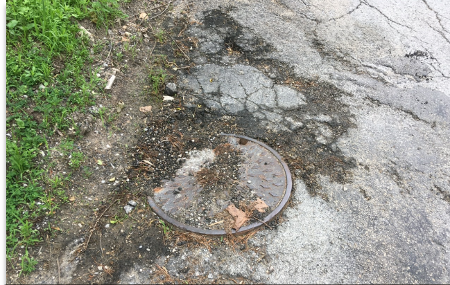
Replacing Sanitary Sewer and Manholes
