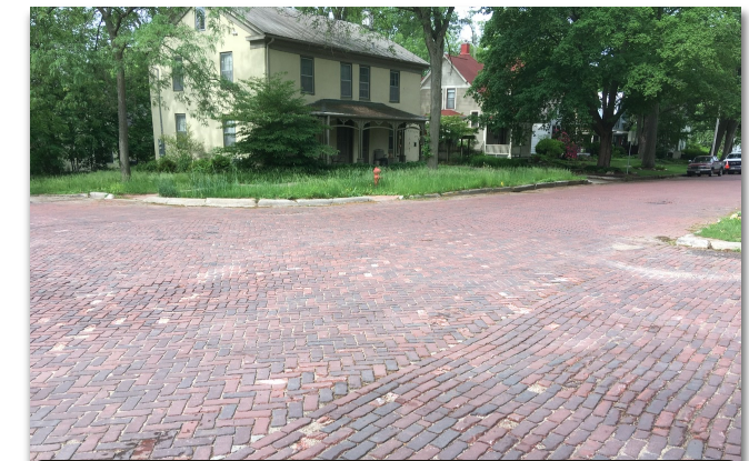
Relay and Preserve Brick Intersection
