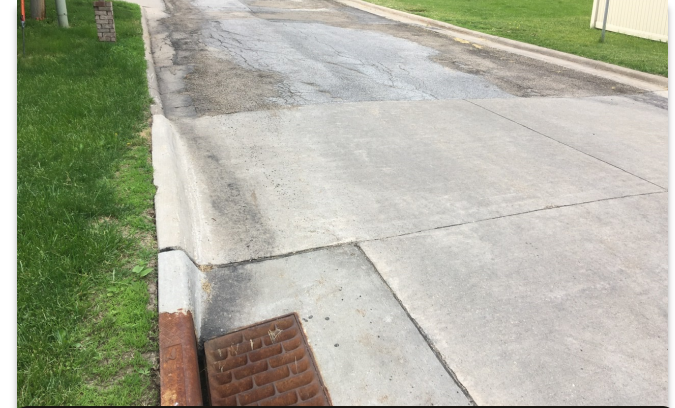
Extending Storm Sewer and Drains
