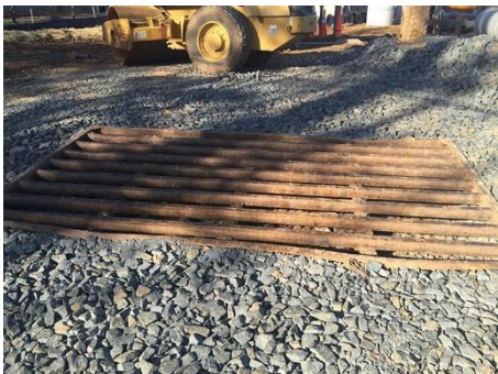
Rumble pad construction exit. Photo credit: John Kosco, Tetra Tech.
