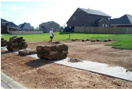
Photo of sod being installed at a residential site. Photo credit: Barry Tanning, Tetra Tech
