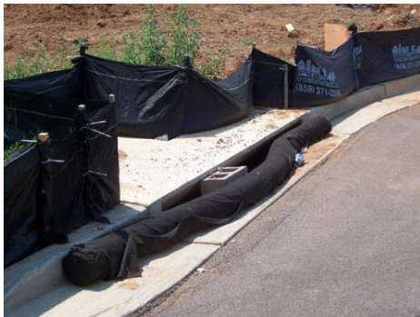
Typical filter bag inlet protection installation. Photo credit: Barry Tinning, Tetra Tech
