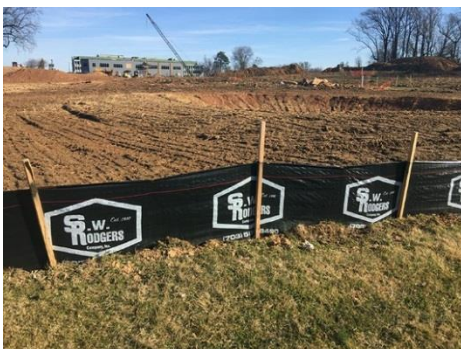
Ensure silt fence is dug into ground to prevent runoff from escaping underneath. Photo credit: John Kosco, Tetra Tech
