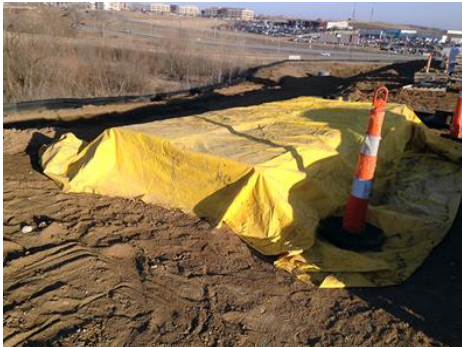
Cover materials using tarps or plastic sheeting to prevent precipitation from contacting construction site materials. Direct work crews to replace material stockpile covers at the end of the day and before rain. Photo credit: Barry Toning, Tetra Tech
