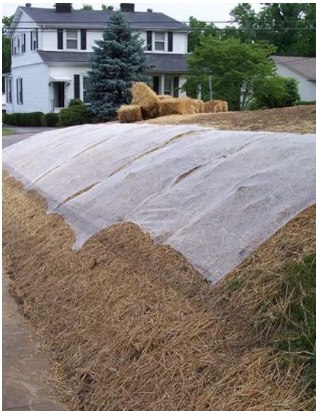
Slope stabilization using mulch and mulch nets. Photo credit: Barry Tanning, Tetra Tech
