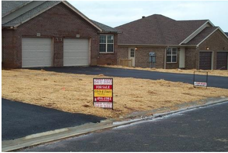
Straw mulch can be used to both prevent erosion and minimize dust from a site. Photo credit: Barry Toning, Tetra Tech.
