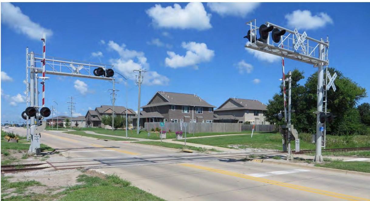
Figure 9: Typical CRANDIC Corridor Active Grade Crossing at Forever Green Road in North Liberty
