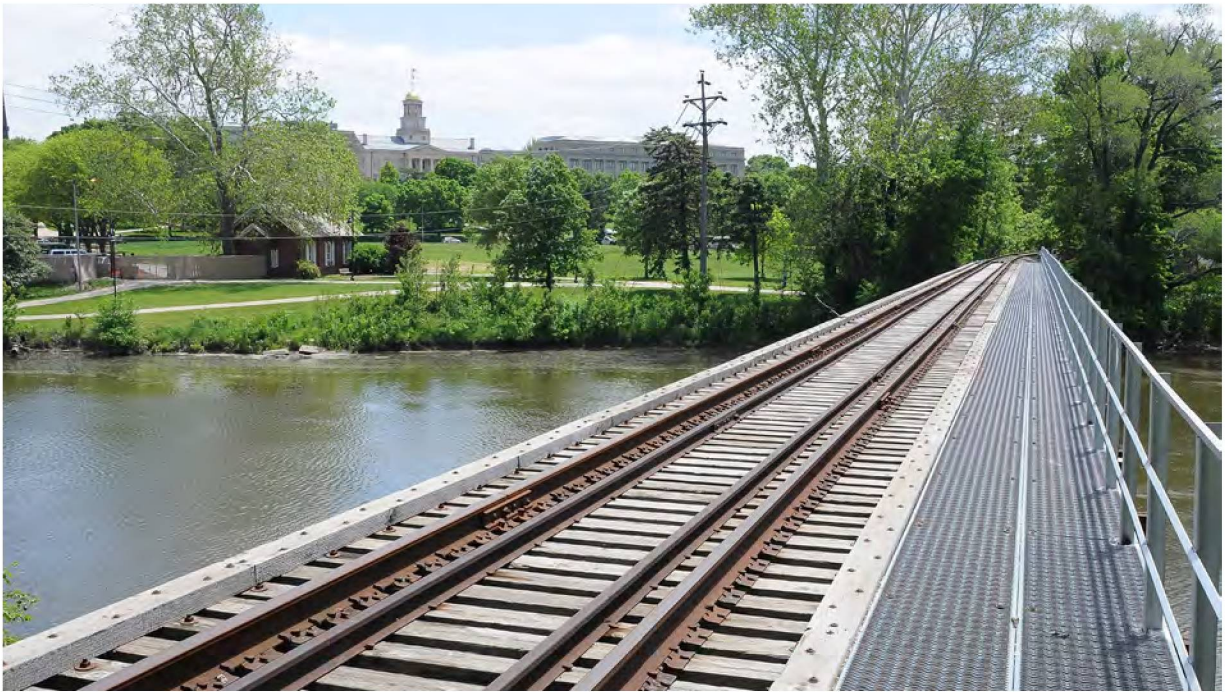
Figure 7: Iowa River Bridge in Iowa City
