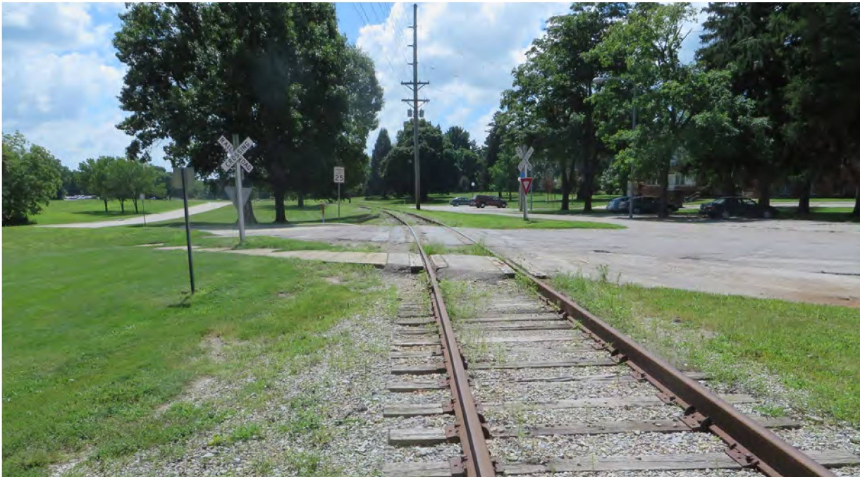
Figure 10: Typical CRANDIC Corridor Passive Grade Crossing at Postal Road in Oakdale
