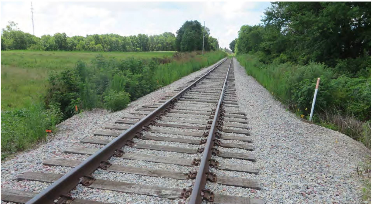
Figure 11: Fiber Optic and Utility Infrastructure in the CRANDIC Corridor near North Liberty
