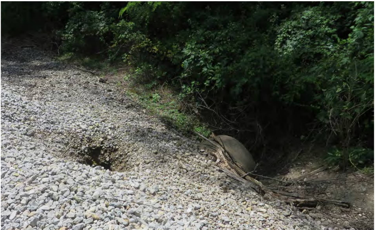
Figure 8: Typical Culvert near Coralville
