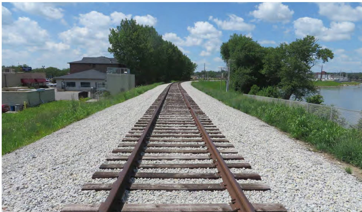
Figure 6: CRANDIC Corridor Main Track Structure in Iowa City
