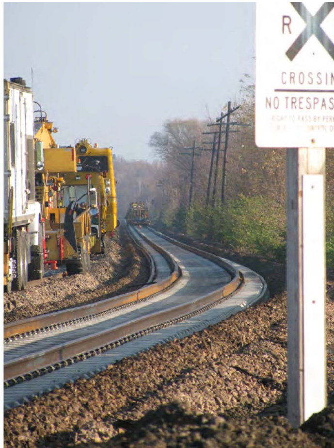
Figure 16: Typical Track Renewal Train with “Skeletonized” Track
