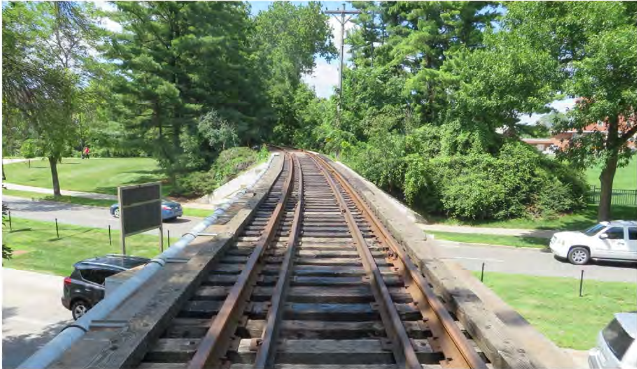
Figure 5: Curvature and Grade on the CRANDIC Corridor at Iowa Avenue in Iowa City
