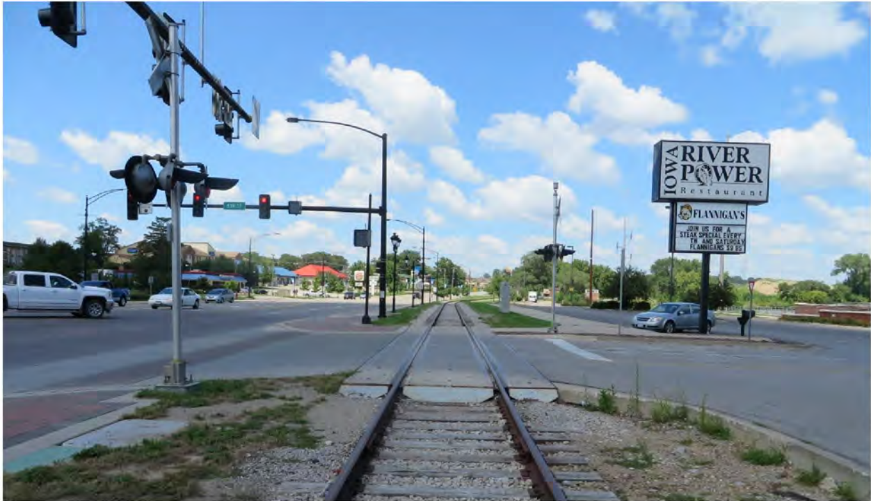
Figure 6: Proximity of the CRANDIC Corridor to Public Roadways at First Avenue in Coralville
