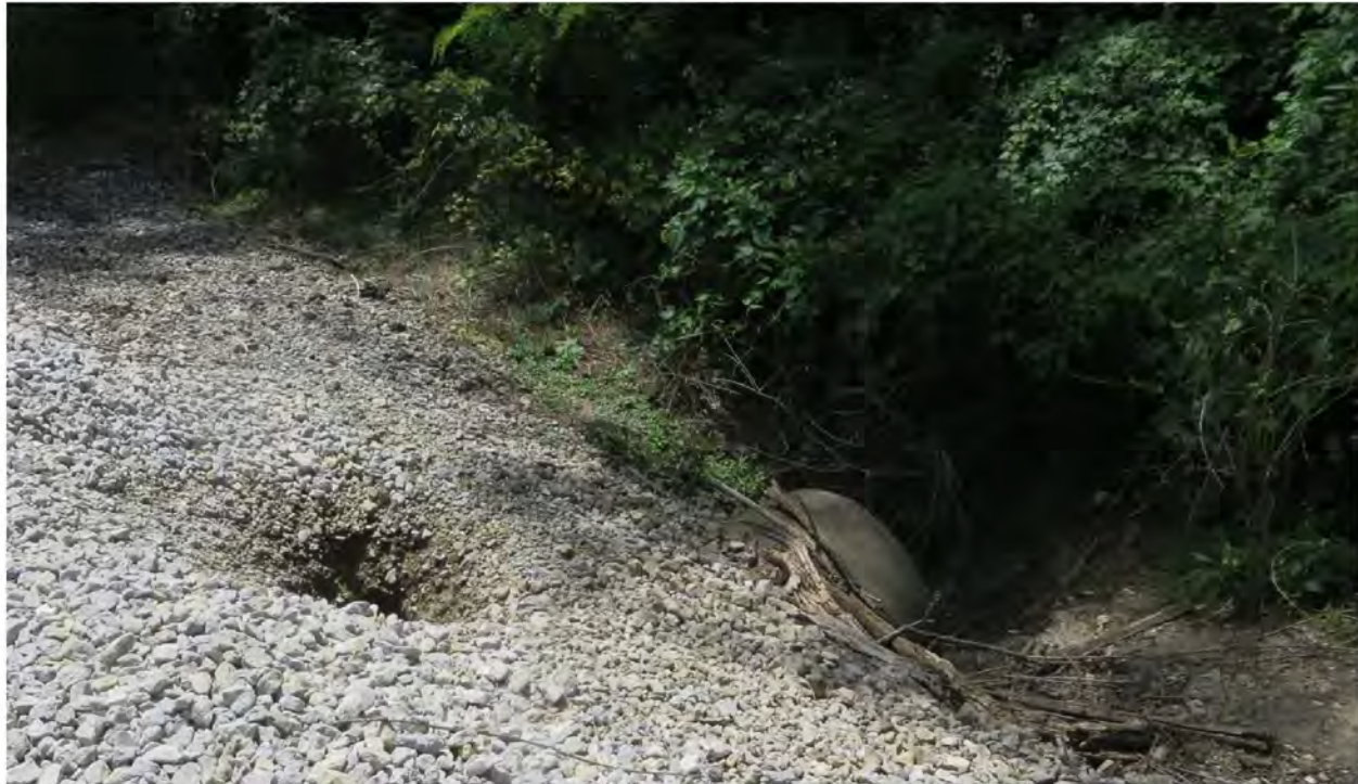
Figure 10: Typical Circular Concrete Culvert (CCP)
