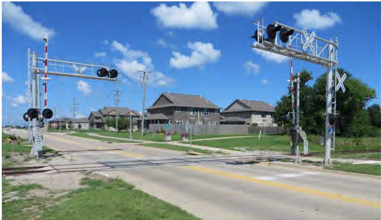
Figure 11: Typical CRANDIC Corridor Active Grade Crossing at Forever Green Road in North Liberty
