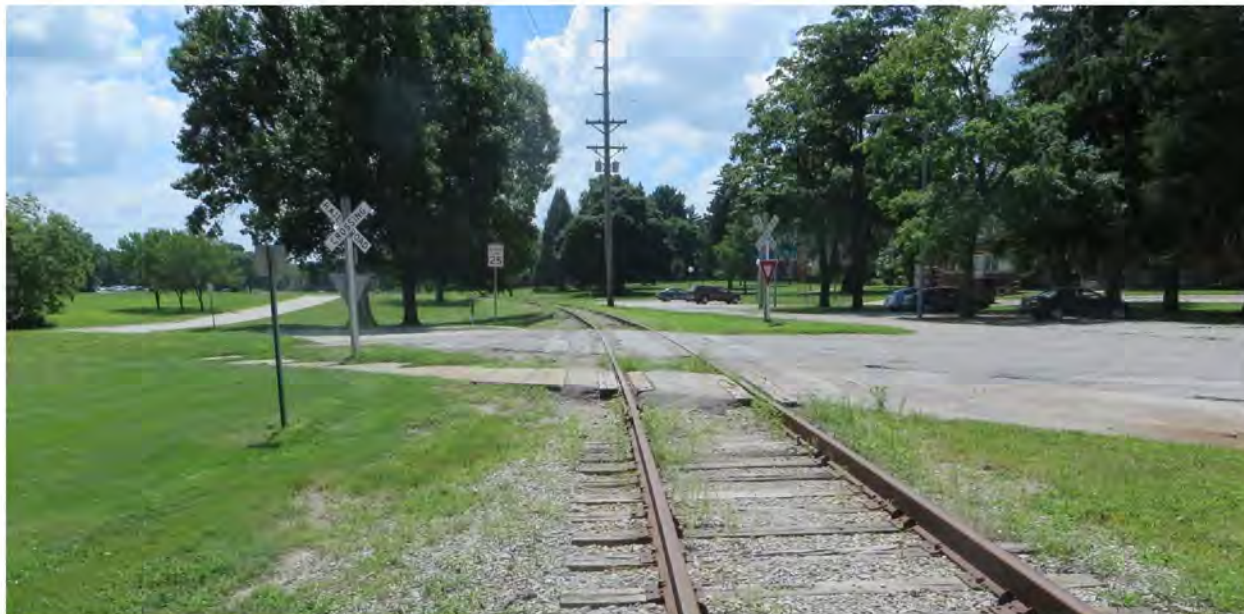
Figure 12: Typical CRANDIC Corridor Passive Grade Crossing at Old Hospital Road in Oakdale
